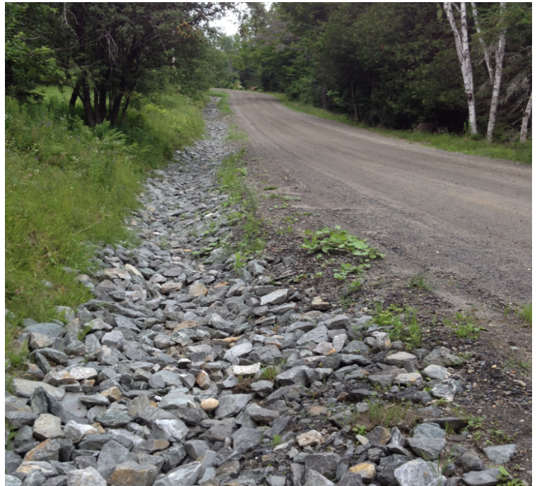
Shadow Lake stone lined ditch. Photo Credit: VTDEC
